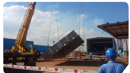
4 inch PLET mudmat being turned over
